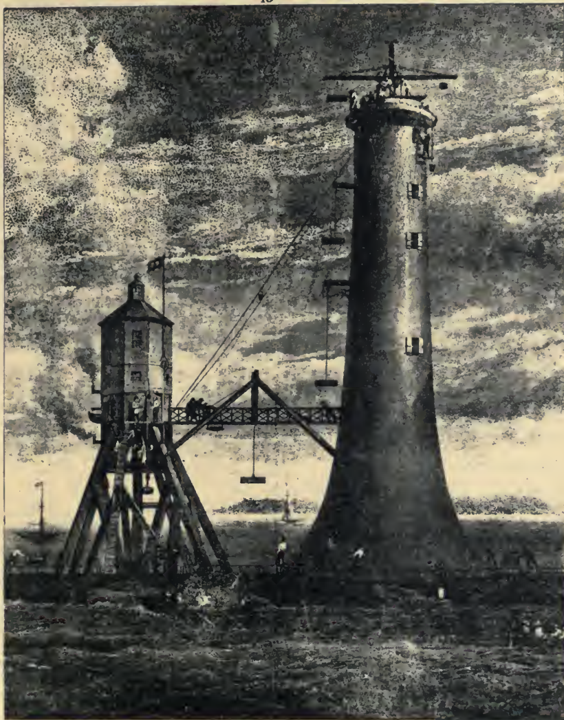
GENERAL VIEW OF THE BELL ROCK WORKS.
